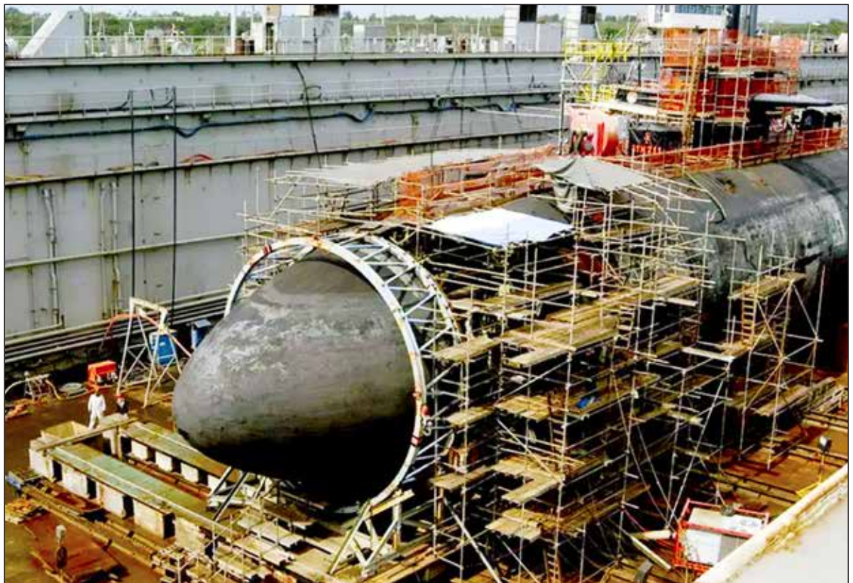
A photo showing temporary repairs made to the USS San Francisco to allow her to sail to PSNS. (U.S. Navy photo.)
